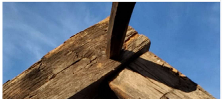
Above: Photo shows original wooden peg joining rafters, taken when schoolhouse roof was reinstalled after the move.
