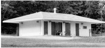
Bassett Shower House
