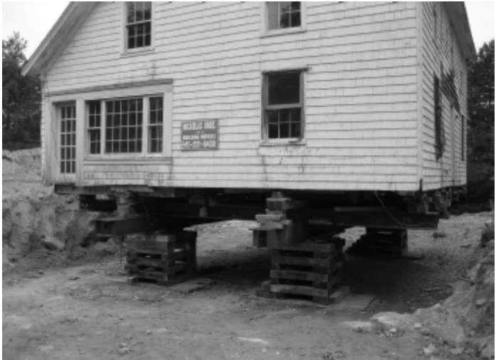
October 11, 2006. The Homestead rests in a trench, supported by I-beams, held in place by blocks of wood, awaiting installation of a foundation and chimney base. (Joy Photo)
